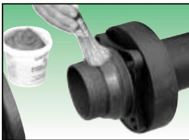
4. Align the bell and spigot for assembly. The ends of the pipes should be in reasonably straight alignment during assembly. Deflections can be made after assembly. Make sure there is no dirt stuck to the lubricant in the bell or on the spigot. Insert the spigot end completely into the bell socket.
