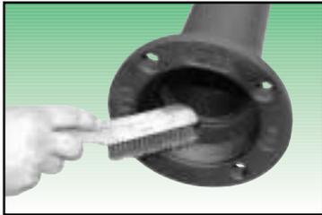
2. Using Griffin pipe joint lubricant, apply a film of the lubricant to the gasket seating area of the bell. Do not assemble the joint without lubrication! The lube allows the MJ gasket to flow into its proper position when compressed by the gland assembly.
