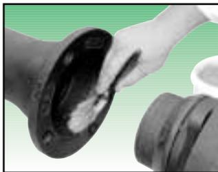
3. Place the MJ gasket over the spigot end of the pipe. Slide the gasket back against the MJ gland. The narrow end of the gasket should face the spigot end of the pipe. Apply joint lubricant to the gasket surface. Do not assemble the joint without lubrication!
