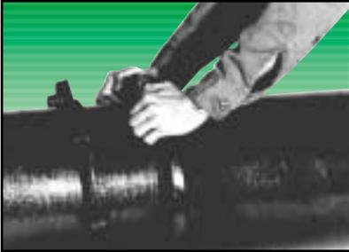
2. Insert the pipe into the socket and press the gasket firmly and evenly into the gasket recess. Keep the joint straight during assembly.
