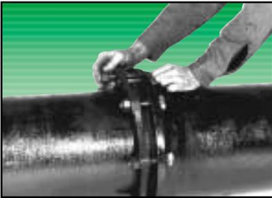
3. Push the gland toward the socket and center it around the pipe with the gland tip against the gasket. Insert bolts and hand-tighten the nuts. Make deflection after joint assembly but before tightening the bolts.
