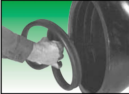
3. Make sure the plain-end is beveled per Griffin Pipe recommendations. Square or sharp edges may damage or roll the gasket causing a leak. The plain-end should be in reasonably straight alignment and carefully guided into the socket. After contacting the gasket, the joint is completed by pushing the pipe until fully seated in the socket. The spigot stripes are used for reference to indicate proper assembly.
