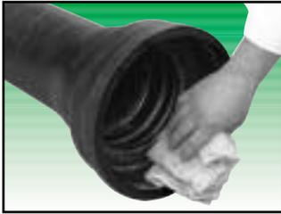
2. The gasket must be wiped clean with a clean cloth. Place the gasket into the socket with the rounded bulb-end entering first. Looping the gasket before the initial insertion will facilitate seating the gasket evenly around the retainer seat. Smaller sizes will require one loop while a larger gasket may require 2 loops. In cold weather (below 40°), the gaskets should be warmed for easier insertion.
