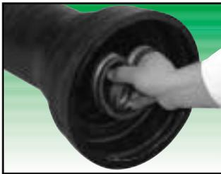
3. Apply a thin film of pipe joint lubricant to the surface of the gasket that will contact the spigot end (plain end) of the pipe.
