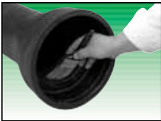
4. Remove any packing material from the pipe spigot. Clean dirt or debris from the outside of the large restraining ring. Clean the spigot end of the pipe and grind or file any sharp edges that may damage the gasket. Apply lubricant to the outside of the spigot end.
